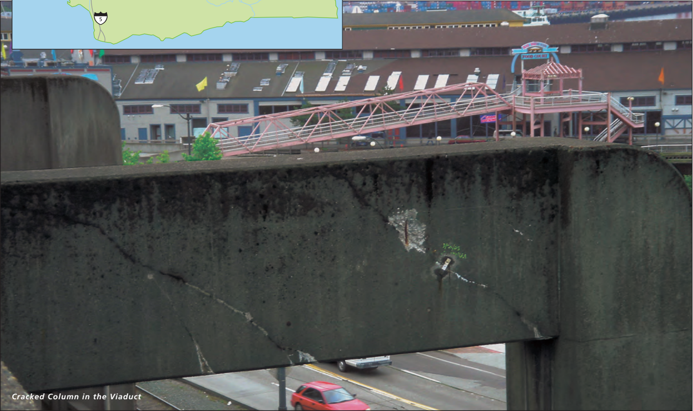
Damaged Rebar in the Viaduct
