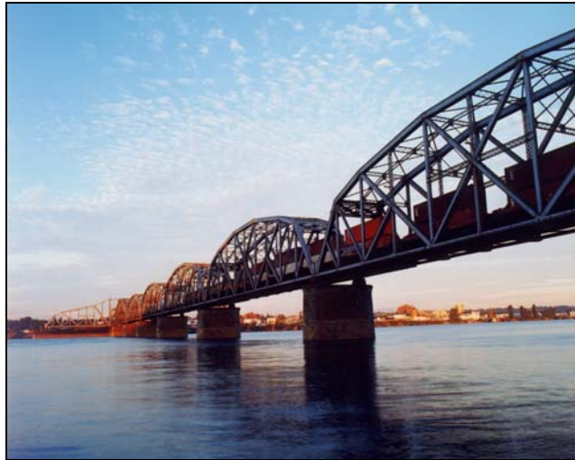
BNSF Columbia River Bridge with open swing span
