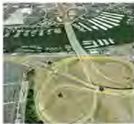
Existing I-5/Marine Drive Interchange
